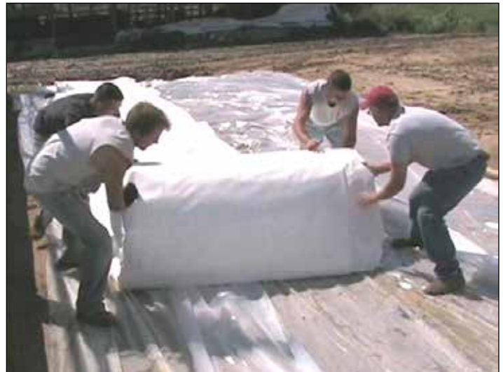
Photo above shows the cover as it is unrolled to prepare for installation. Cover is heavy. Assistants are required.
