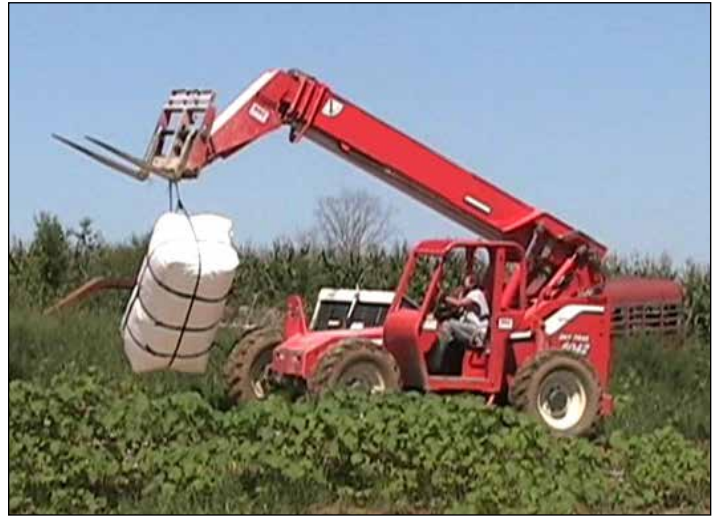
Photo shows moving the cover prior to preparation and installation.
