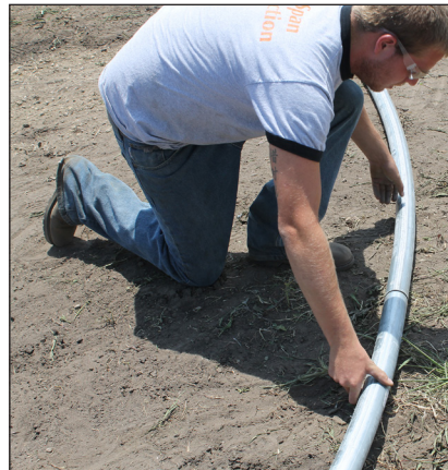
STEP 1: Connect rafter pipes. Actual rafter pipe and connection may differ.
