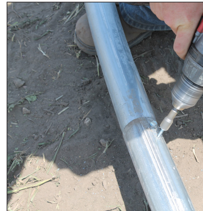
STEP 2: Secure each rafter joint using two (2) FA4482B Tek screws.
