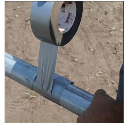
STEP 3: Wrap each splice and Tek screws with 115198 duct tape to protect the film cover.
