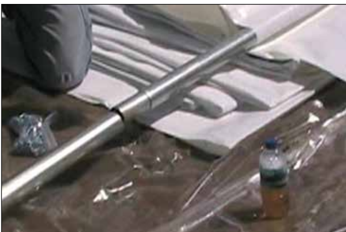
Photo shows connecting first two pipes.
