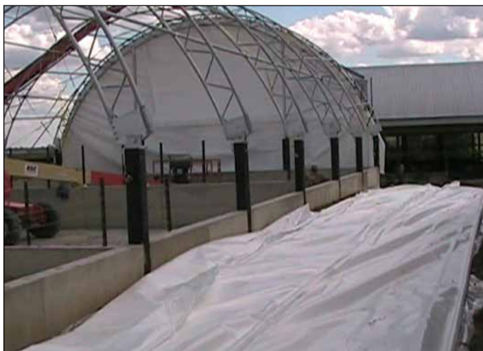
Photos show cover as it is unrolled to prepare for installation. Cover is heavy. Use assistants to unroll and prepare.
