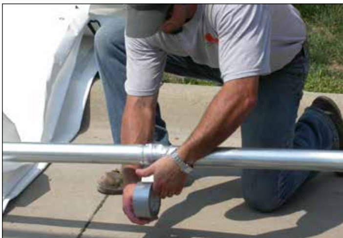
Wrap splice and Tek screws with duct tape.
