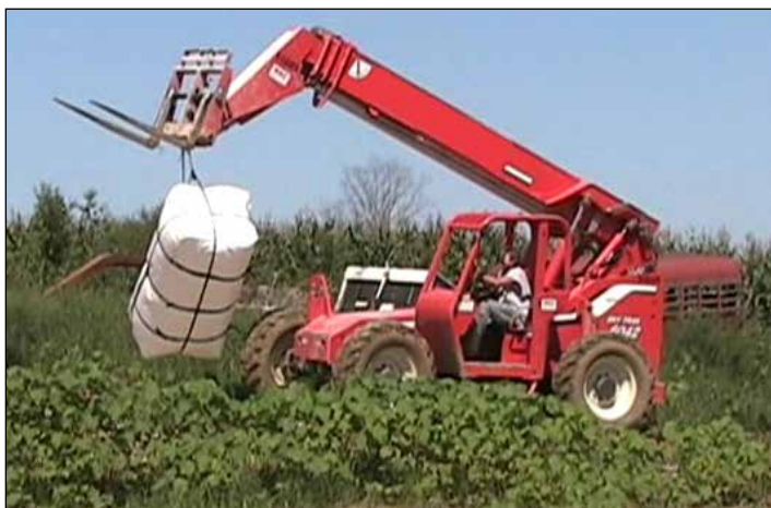
Photos show cover as it is unrolled to prepare for installation. Cover is heavy. Use assistants to unroll and prepare.
