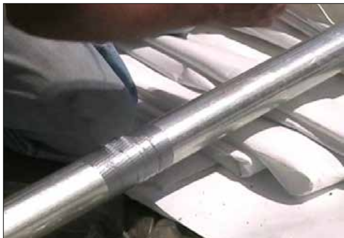
Wrap splice and Tek screws with duct tape.
