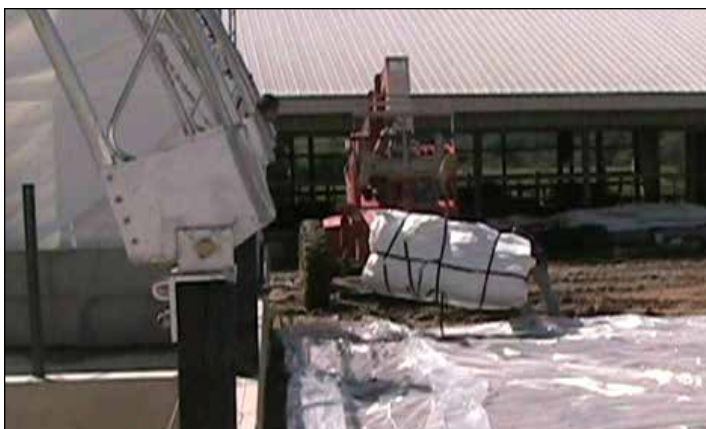
Move cover to prepare and install. Set into position next to frame.
