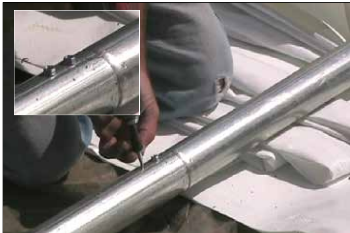
Install two Tek screws to secure each pipe joint.
