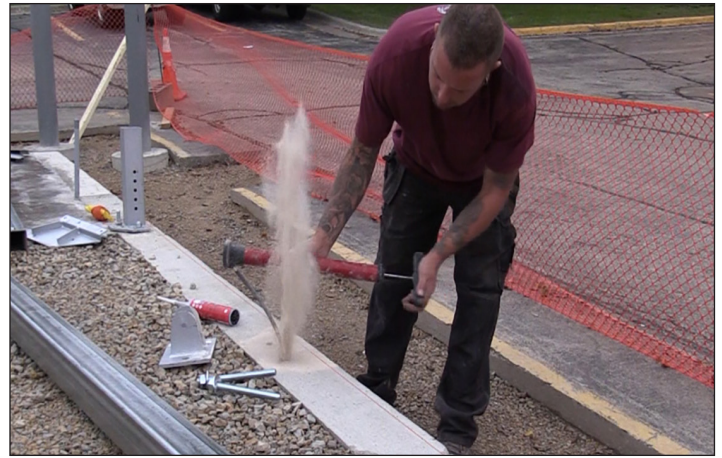
STEP 6: Clean out the hole.
