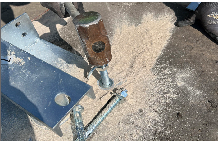
STEP 8: Hammer wedge anchors into holes.
