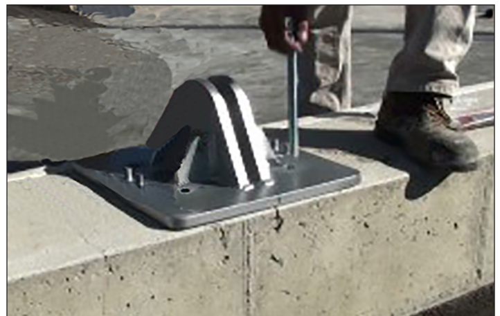
STEP 7: Install wedge anchors.
