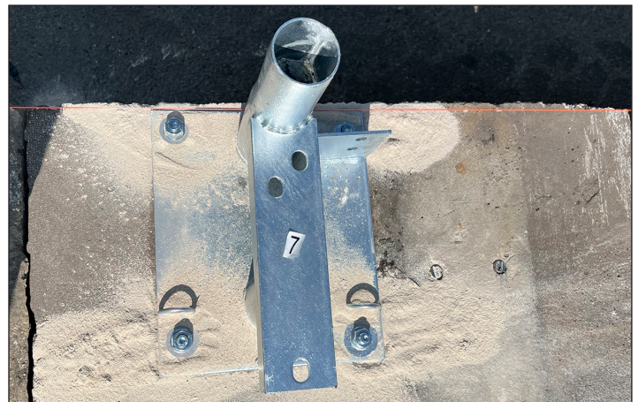
STEP 10: Hand tighten all nuts.
