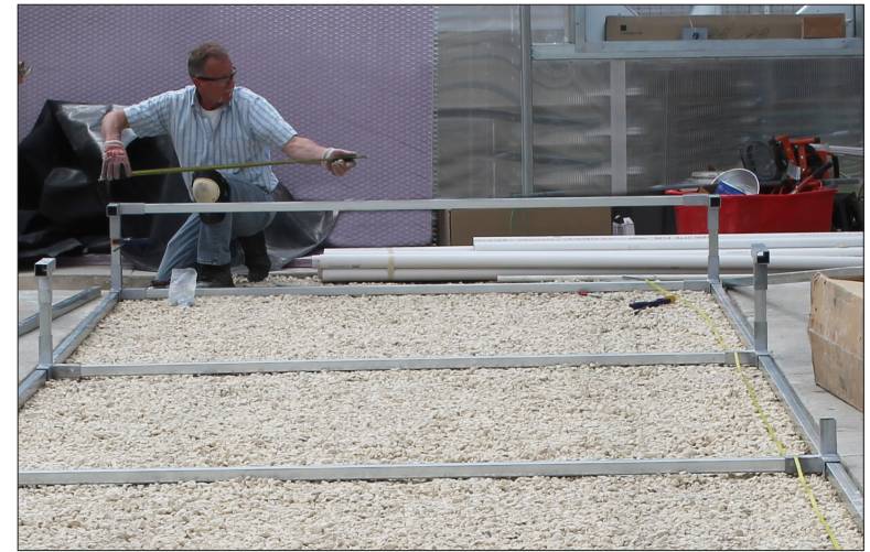
Above photo shows assembled cross supports installed and spaced on lower perimeter frame. Cross bed supports are supplied on models 115331 thru 115335.
