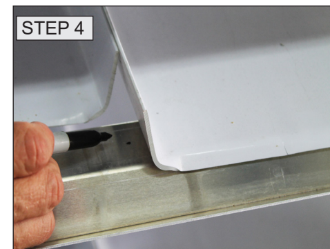
Center fastener location so screw head does not contact any part of any tray.
