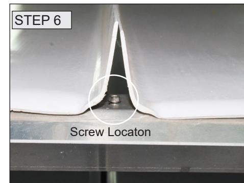
Photo shows trays in position with fastener installed to secure gutter.
