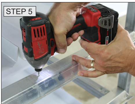
Slide trays back from gutter to allow for the installation of the 112838 fasteners.
