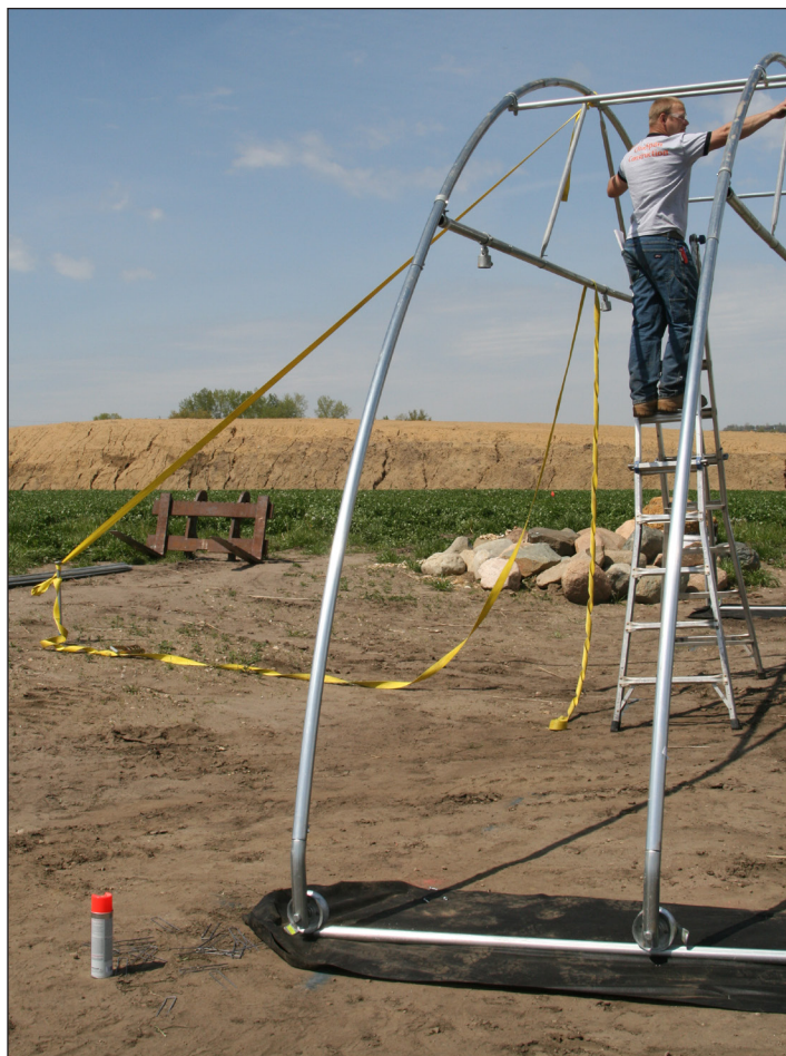
Photo shows the first end rafter and first interior rafter set in place on the track pipe. End rafter is secured to the site using one of the anchor stakes included with the building.
