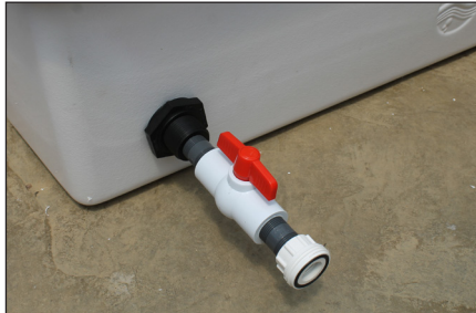
Attach section A to bulkhead fitting.
