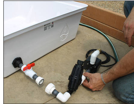
STEP 4: Disconnect pump assembly from reservoir.
