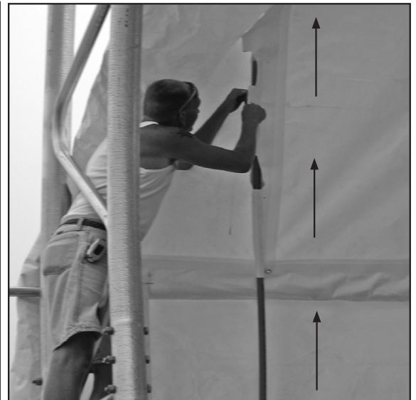
Photo shows the notched stretch pocket and the installed PVC conduit at the end of a similar main cover.
