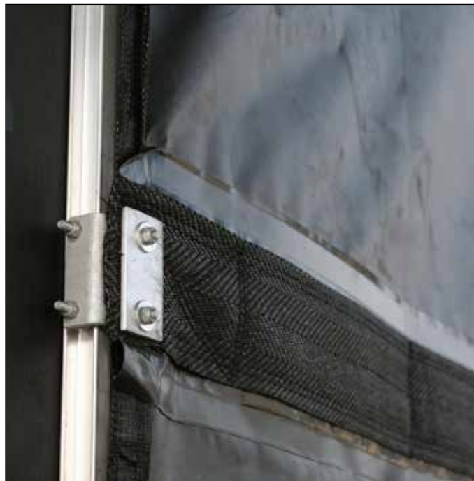
Photo above shows bearing plate and door panel as seen from inside the building.
