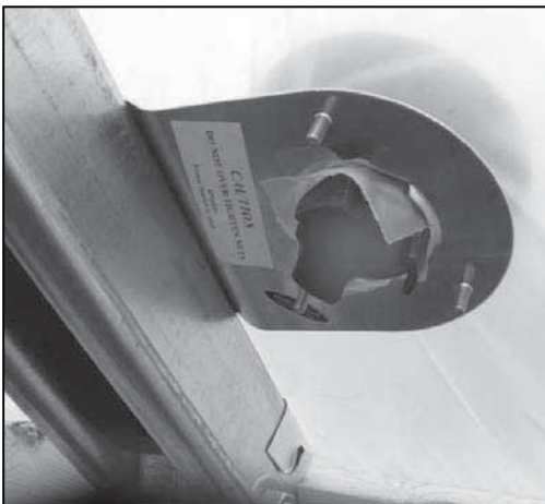
Inside view showing fan mounting bracket and the mounting bolts for the fan.
