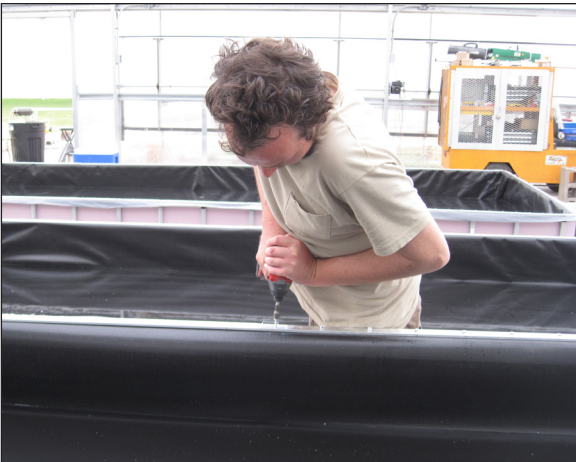
Photo above shows installing aluminum bar and Tek screws to secure liner.
