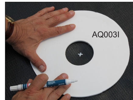
d. Align center of support washer with center mark.
