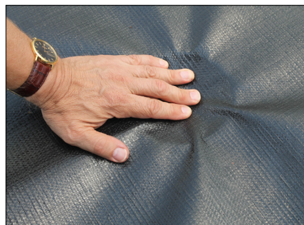
a. Lightly press liner to reveal outline of hole.
