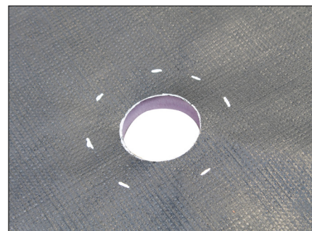
i. Check position and remove loose material.
