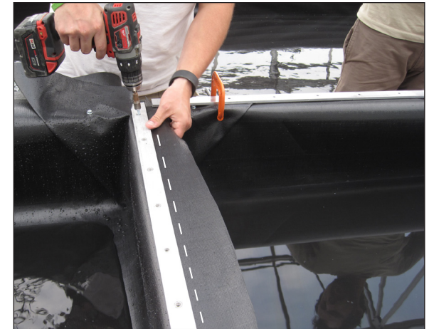
Photo shows securing adjacent liners to same crossbar. Trim liner material as needed once material is secure. See dashed line above.
