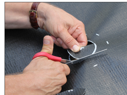
h. Use a scissors to cut fitting hole in bed liner.
