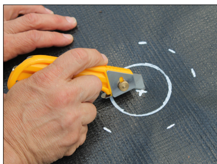
g. Use a utility knife to carefully cut center mark.
