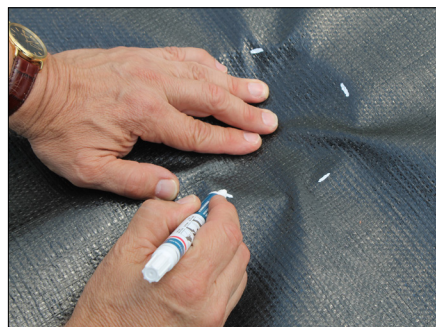
b. Mark hole using a paint marker or similar tool.
