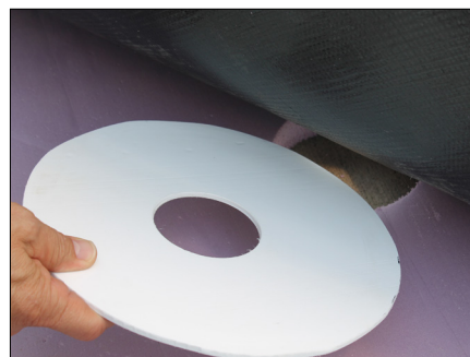
k. Slide support washer between liner and insulation.
