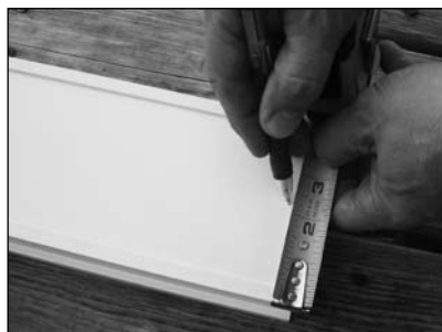
Find center of channel bottom.
