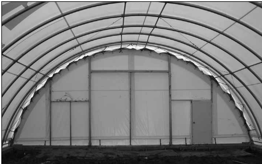
Photos show end panel examples. Lower photo shows an installed panel as seen from the inside.
