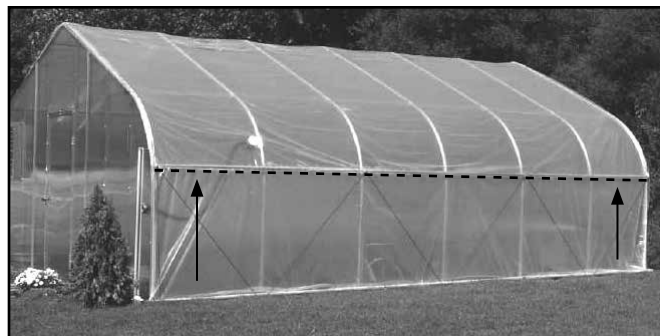
Attach main cover to Poly Latch U-Channel.
