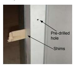
Cut the shims flush with the inside and outside of the jamb.  Follow the instructions that came with the building to install the siding or covering on the building. Siding or covering can be installed up to or overlap onto the door jamb.
