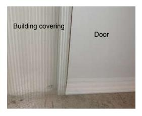
11. Install trim over the siding or covering and door jamb for a weather tight and finished appearance.
