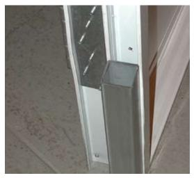
Place wood shims between the door jamb and the frame to square the door in the opening. The shims should be near the pre-drilled holes in the jamb.
